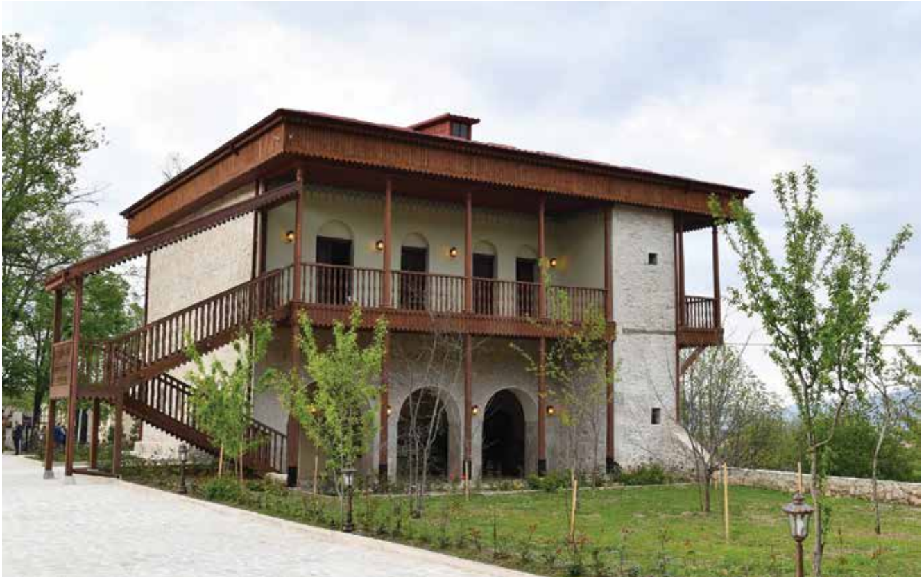
House of the Mehmandarovs after restoration. 2023
